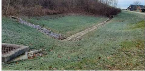
Basin has been modified to hold stormwater during heavy rain events
